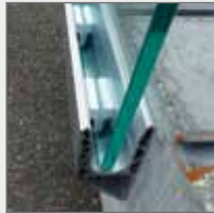
Install the glass
