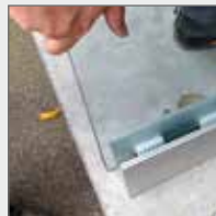
Install the glass
