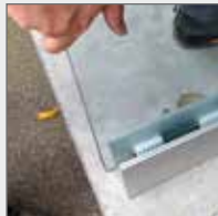
Install the glass
