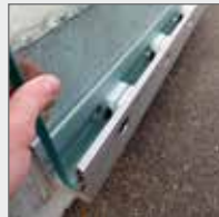
Install the glass
