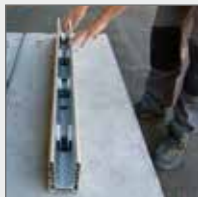
Install the U wedges
