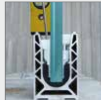
Simultaneously adjust vertical alignment and tighten clamp
