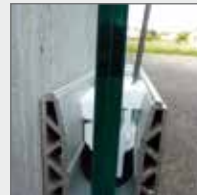
Simultaneously adjust vertical alignment and tighten clamp
