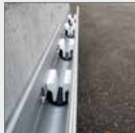
Install the U wedges
