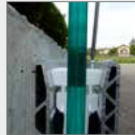
Simultaneously adjust vertical alignment and tighten clamp
