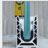
Simultaneously adjust vertical alignment and tighten clamp
